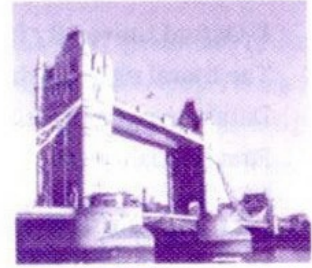
Tower Bridge, London, England
